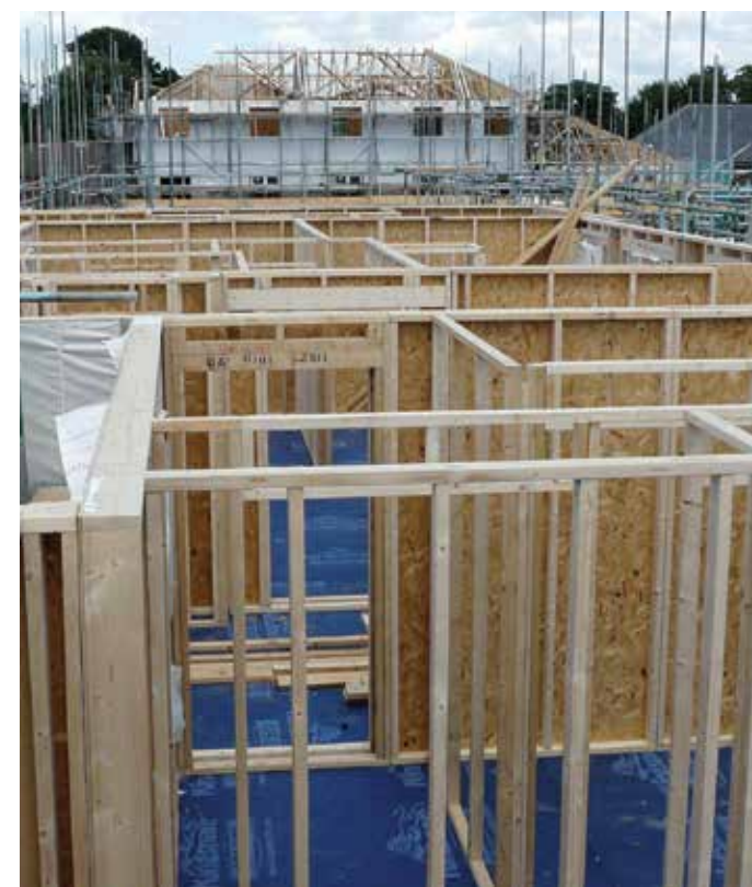
Below left Timber frame built by Robertson Timber Engineering being assembled on site Below right External steel-frame wall panel after being injected with fire-retardant EPS
