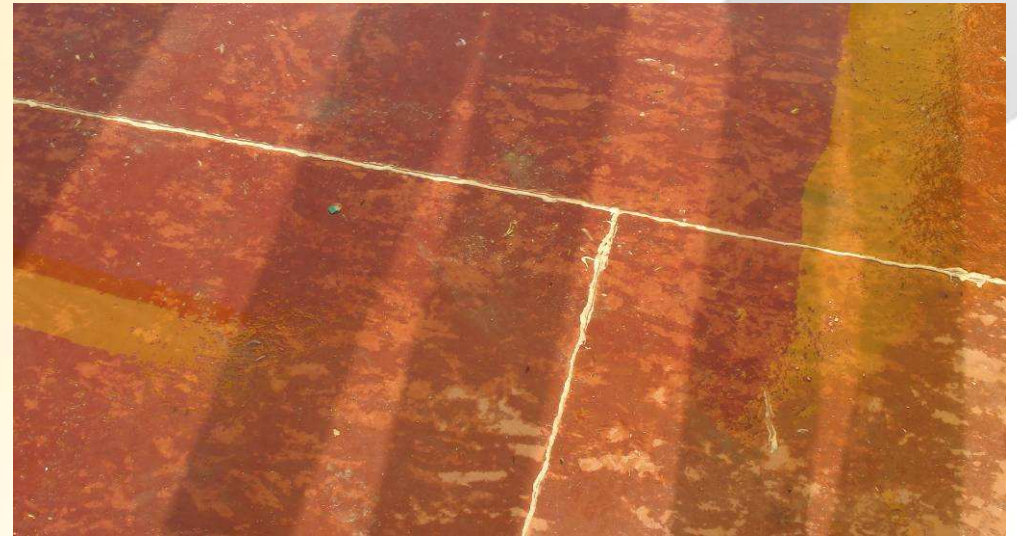
A temporary water proof ply board was laid on top of each floor slab to prevent water penetrating through and staining the exposed CLT panels below. This was removed before the floor screed was laid.
