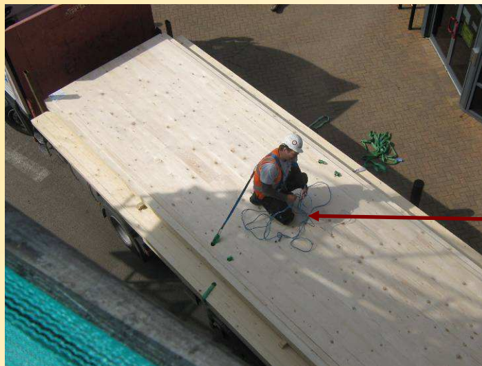
An operative harnessed to a pre-installed lifting strop whilst the crane lifts and positions the previous panel.
