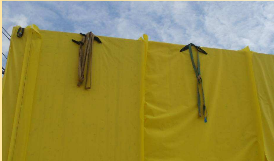
A thin fabric sheet is used to protect CLT panels from sunlight bleaching and other trades on site.
