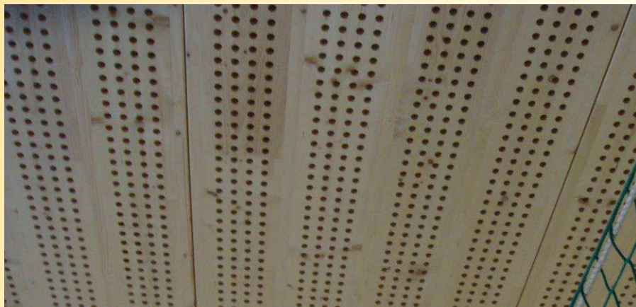
Acoustic relief to the underside of the floor cassette panels (forming the ceilings) provided acoustic attenuation.
