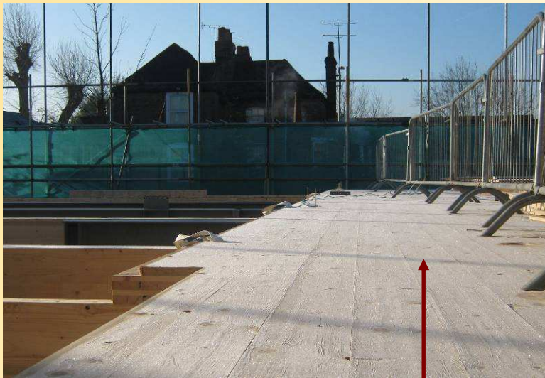
Fixed safety barriers positioned 1m from the leading edge.
