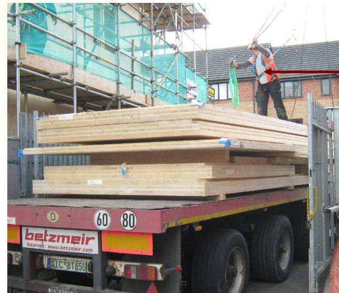
An operative harnessed to a pre-installed lifting strop whilst the crane lifts and positions the previous panel.
